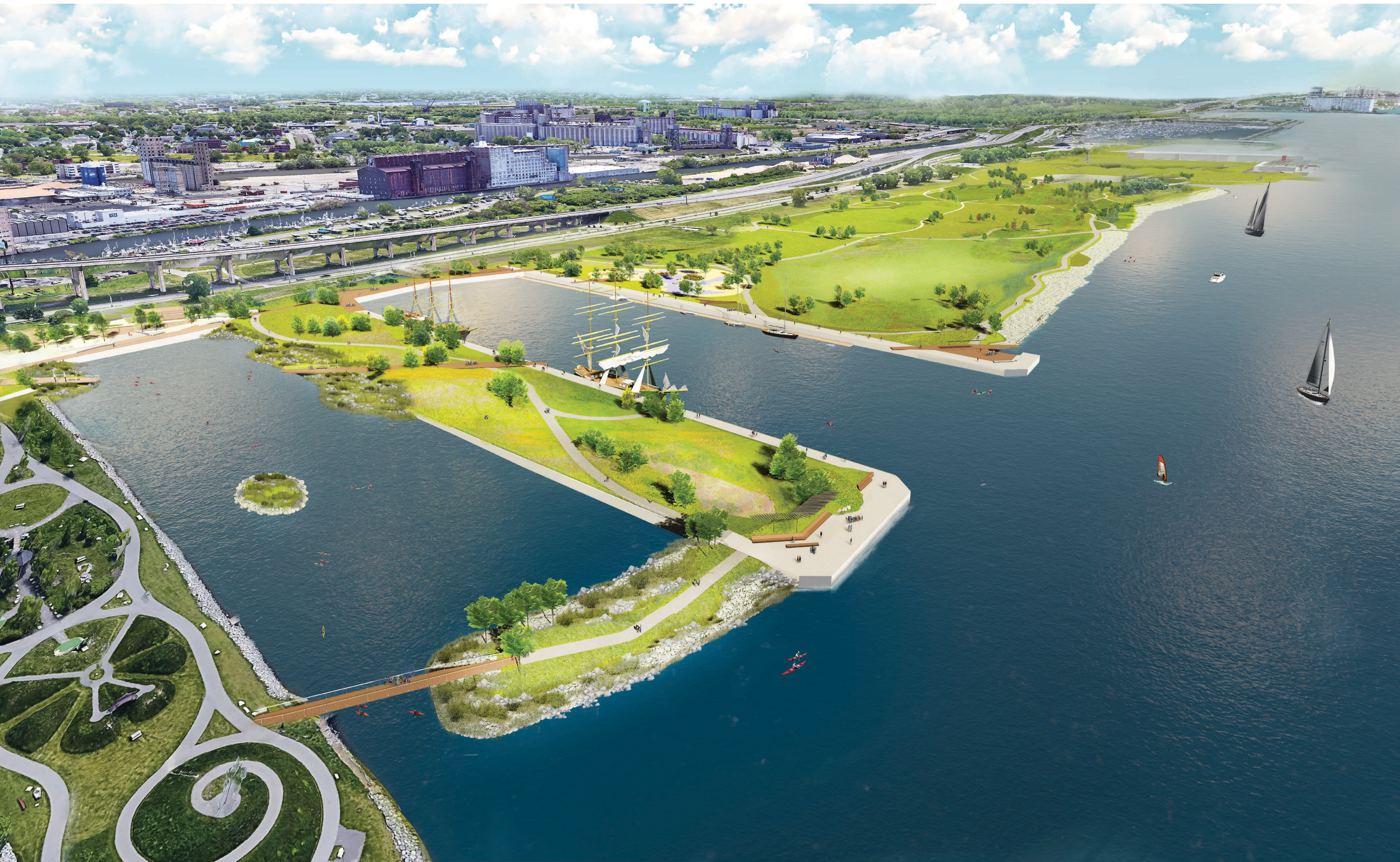
AERIAL VIEW LOOKING SOUTH
