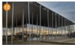
Figure building under roof structure
