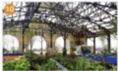
Interior pedestrian courtyard
