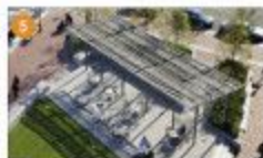
Southern plaza with pavilion
