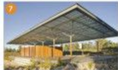
Northern plaza with comfort station and pavilion
