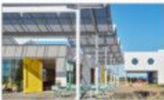
Figure building under roof structure
